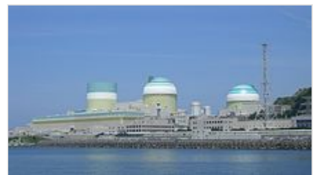
The Ikata Nuclear Power Plant, a pressurized water reactor that cools by utilizing a secondary coolant heat exchanger with a large body of water, an alternative cooling approach to large cooling towers
