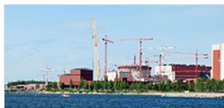
Olkiluoto 3 under construction in 2009. It was the first EPR , a modernized PWR design, to start construction.
